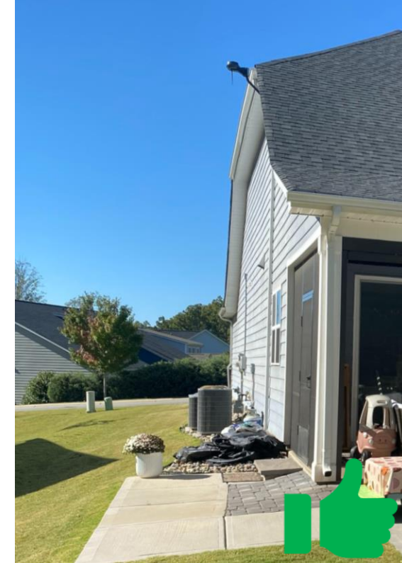
On side of house using a Satellite/Star Link mount to ensure that dome is above the roof line.
